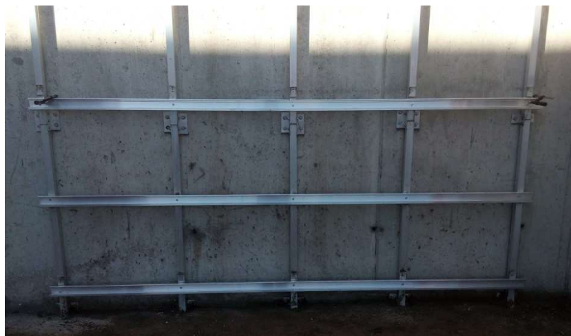
Figure 2.2.16 - View of the rail profile arranged horizontally
